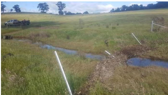
Figures 10-12. Repairing flood damage during Spring 2023
