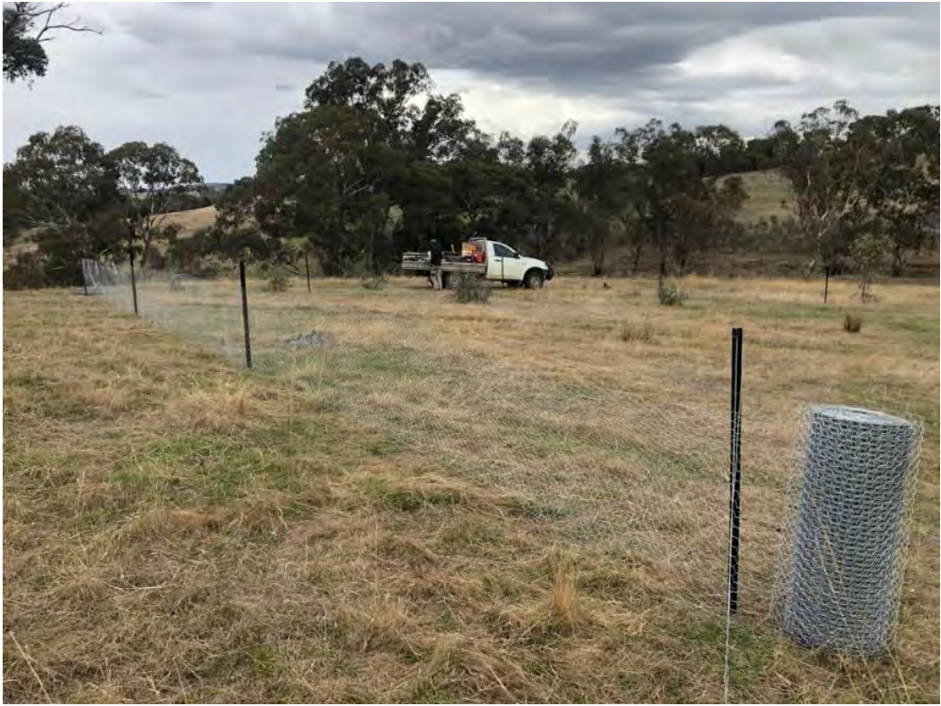
Figure 2. Constructing fence around sheep exclusion zone (control plot); April 20, 2021
