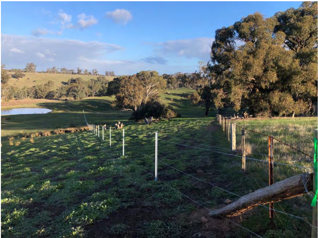
Figure 3. Constructing fence near dam; June 4, 2021
