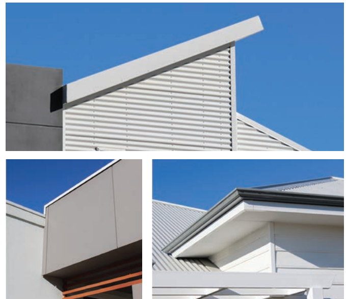
Fig. 15: Typical example of light weight cladding materials.
