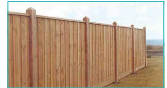
Timber paling fence with exposed posts
