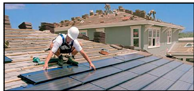
Roof integrated photovoltaics replacing roof material
