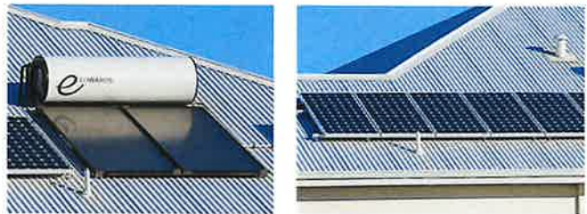
Fig.29:Typical example of solar collectors matching roof profile.
