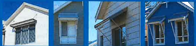
Fig. 20: Typical examples of shade devices over windows.
