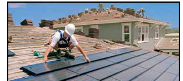
Roof integrated photovoltaics replacing roof material
