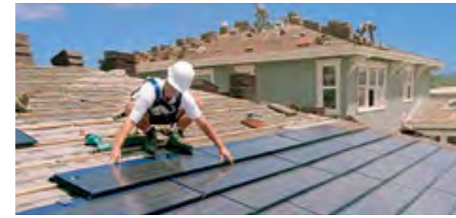
Roof integrated photovoltaics replacing roof material
