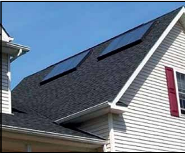
Roof-mounted solar heating
