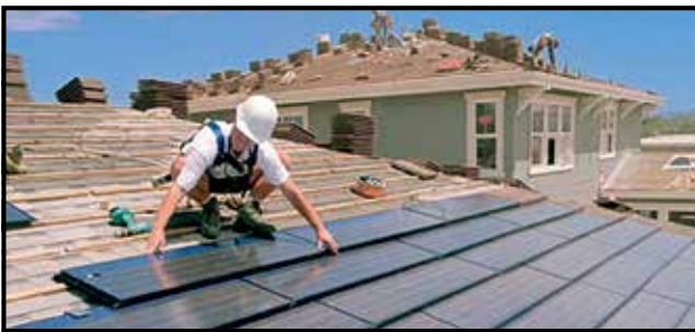
Roof integrated photovoltaics replacing roof material
